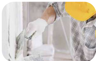
4. Apply the first layer, the thickness is about 1.5mm
